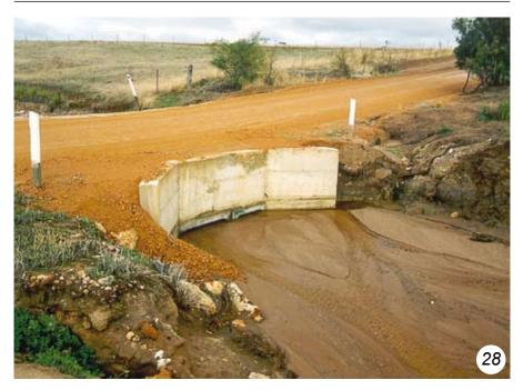
been washed out. However, the weaker foundations of the channel banks have suffered the full impact of the redirected flow, resulting in a new channel.
