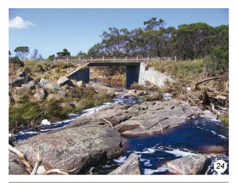
bridge design. The height of the bridge maintains the crosssectional area of the channel and concrete supports are winged, which assists in guiding the flow under the bridge. The winged supports also help armour the banks.
