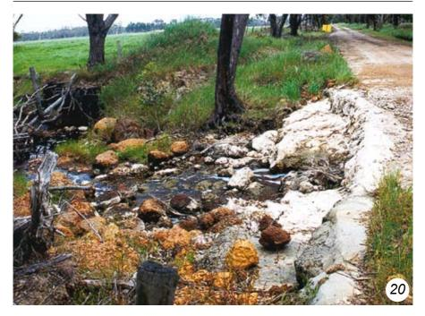
small culvert pipe, which ensured that the 'dam' was regularly overflowing. After many years and quick-fix repairs, the entire crossing was removed and rebuilt using box culverts with a capacity near that of the natural channel.
