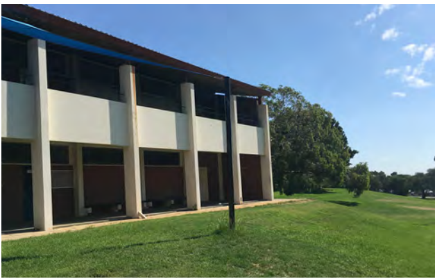
Existing built form/landscape interface
