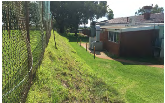
Existing topography, interface between built form and soccer pitch
