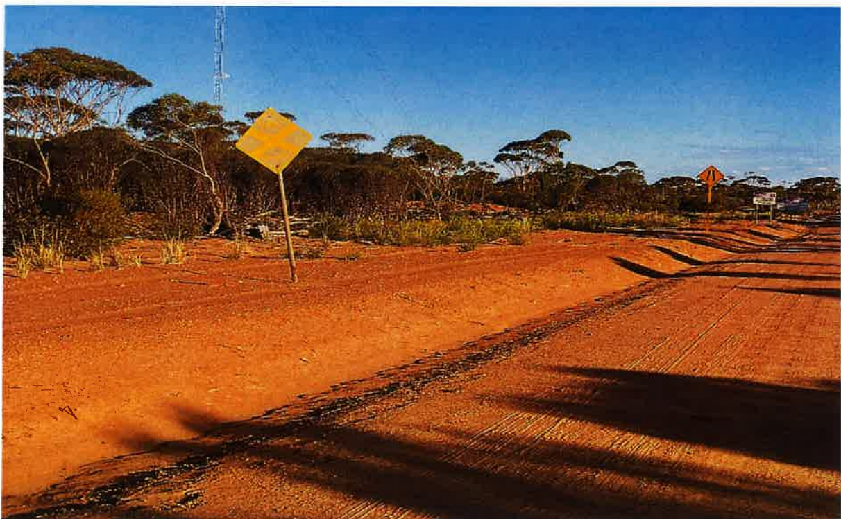
Faded railway crossing sign on north side of railway line
