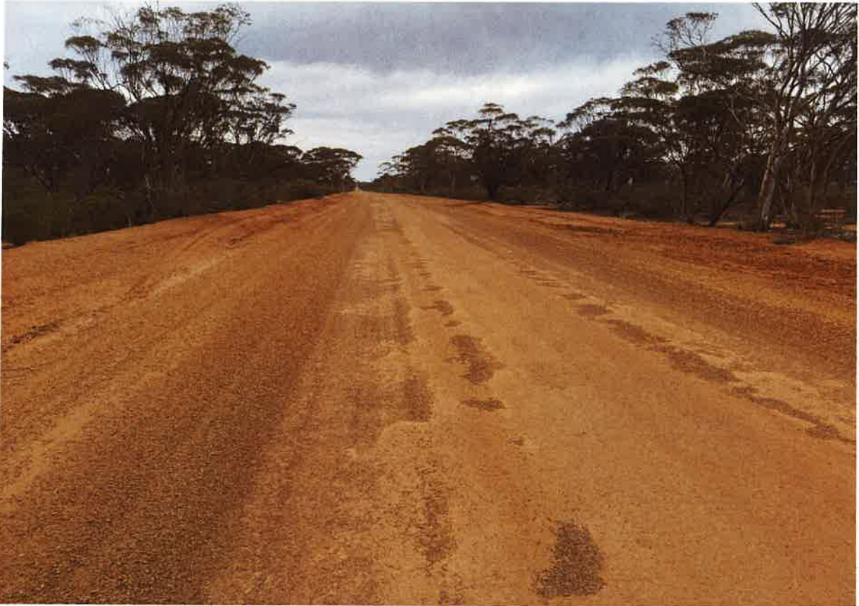
Gravel sheeted section in generally good condition – some minor shallow potholes
