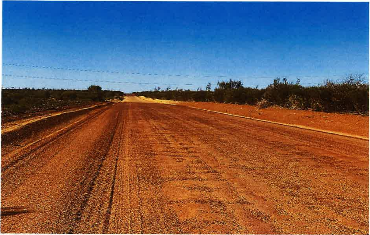
View of road at about 5km mark showing minor corrugations
