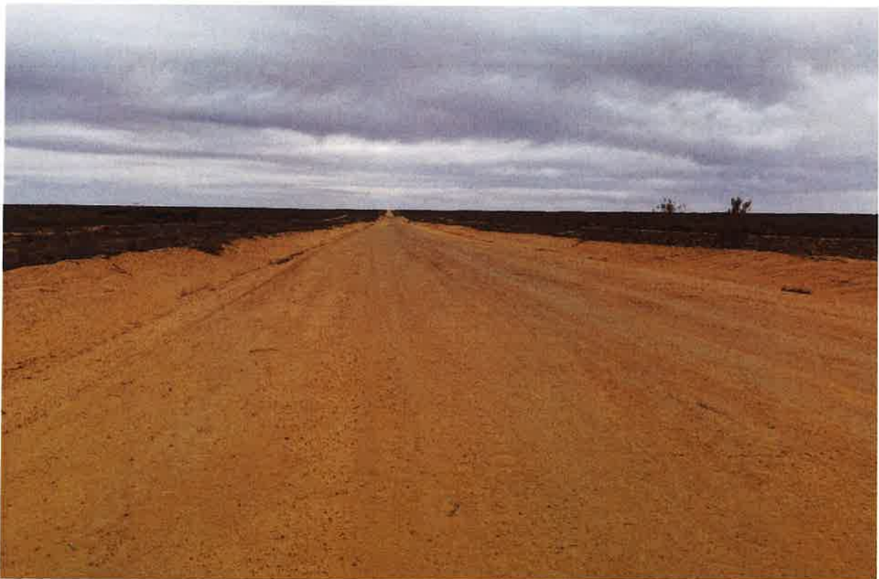
Typical section south of railway line – good condition
