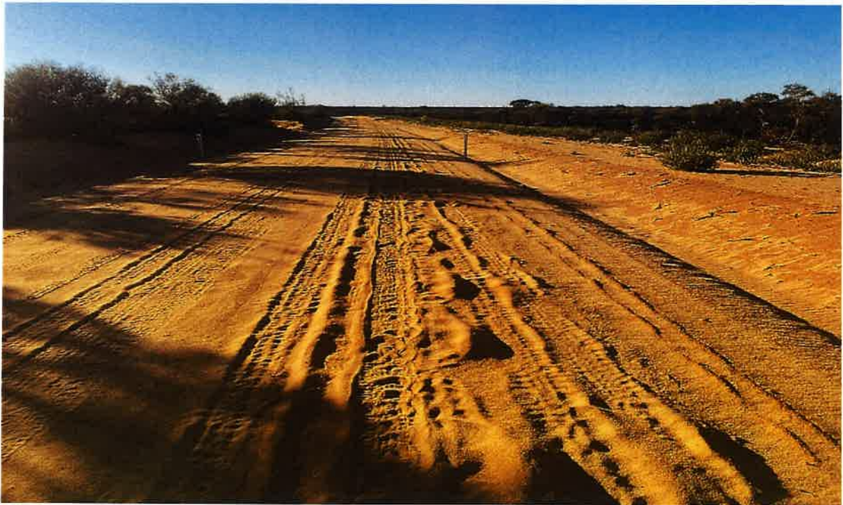
Minor rutting and corrugations in sandy section 2km north of railway line
