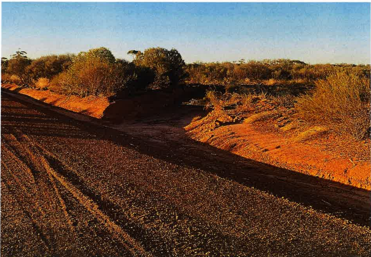
Water lying in deep pit at terminus of wide offshoot drain
