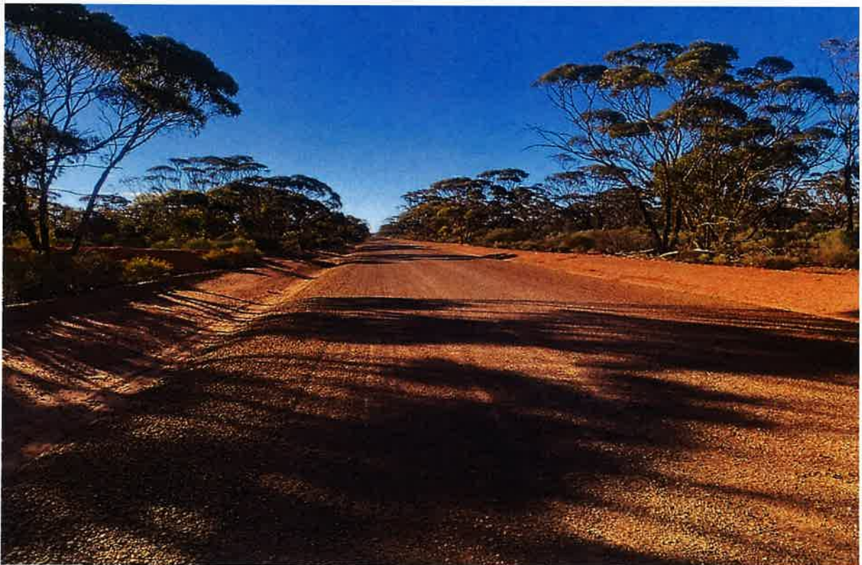
Very smooth section of road at around the 10km mark
