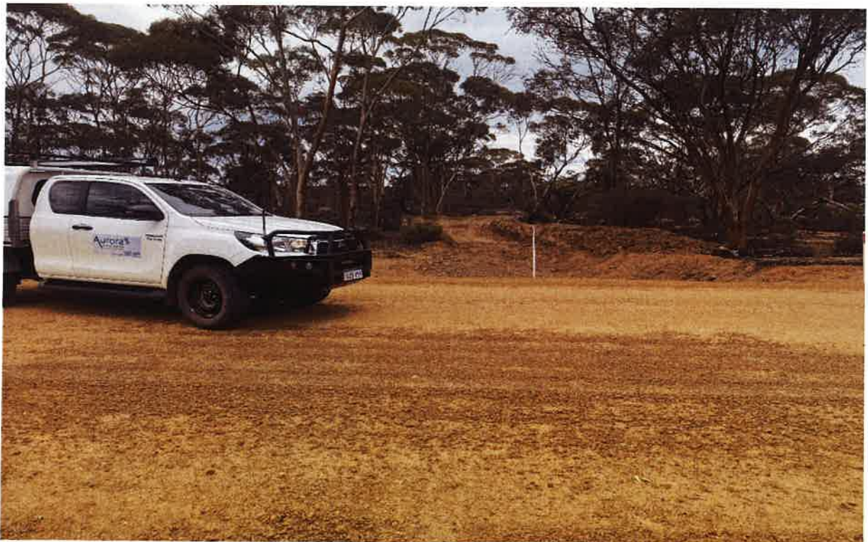
Gravel sheet over sandy section, surface in good condition
