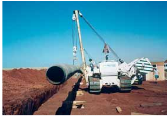
Figure 7.7 Overland Pipeline Installation (Image courtesy of CEIS).
