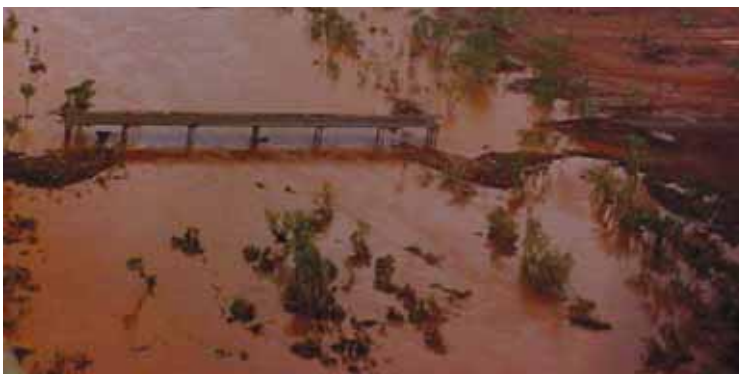
Figure 7.19 Bridge over the Maitland River (Image courtesy of Main Roads WA).
