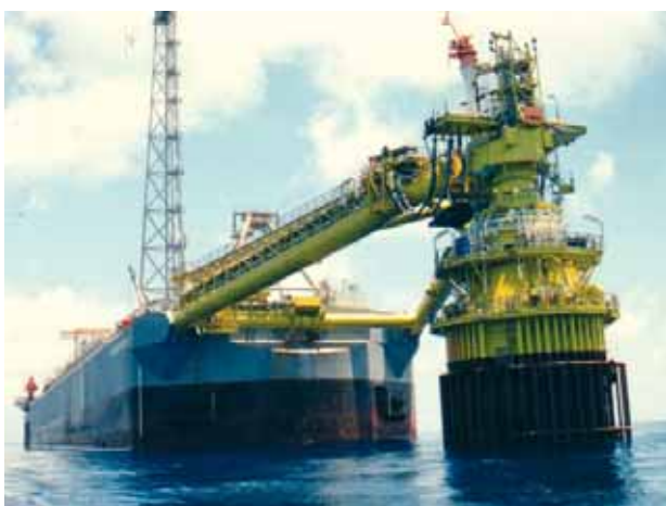
Figure 7.22 Single Point Mooring Facility (Image courtesy of CEIS).
