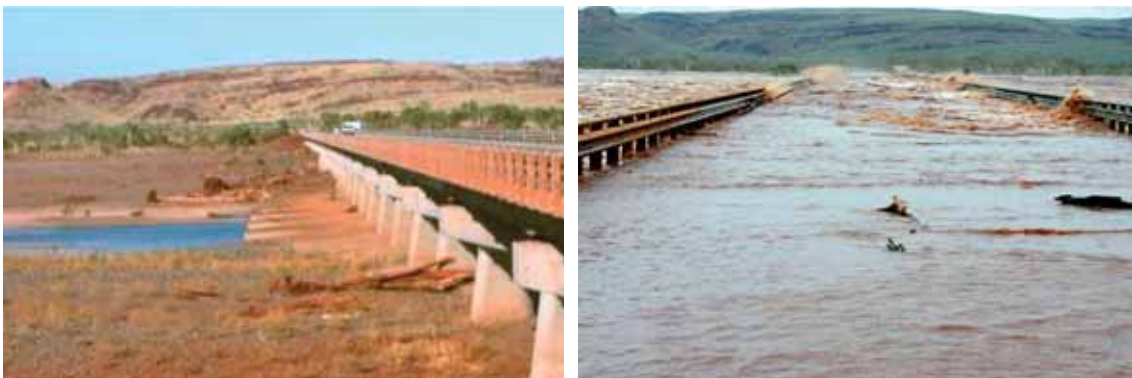
Figure 7.16 Bridge over Fortescue River - in the dry and after Cyclone Monte (Image courtesy of Main Roads WA).
