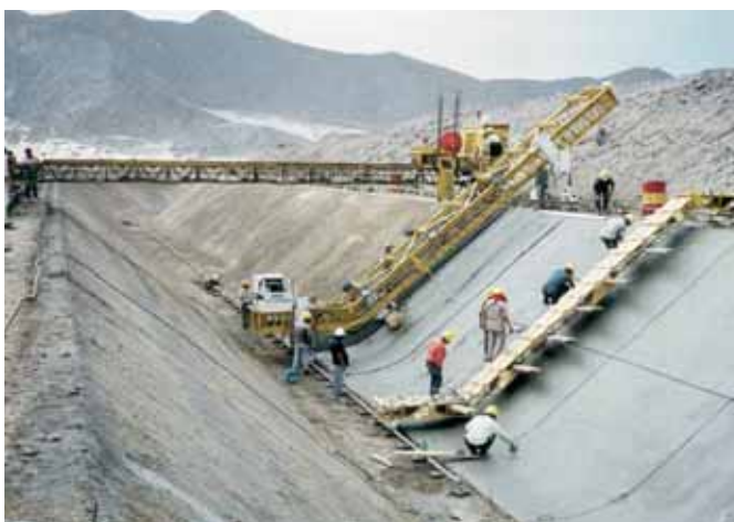
Figure 7.14 Photo of a typical canal lining operation (Image courtesy of GHD).
