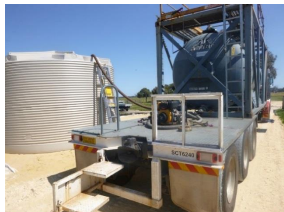
Figure 5: Delivery of clay to the storage tank.
