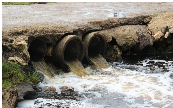
Figure 2: A pipe culvert 20 m downstream of the clay dosing site.
