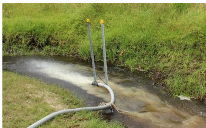
Figure 7: Clay application to the drain.
