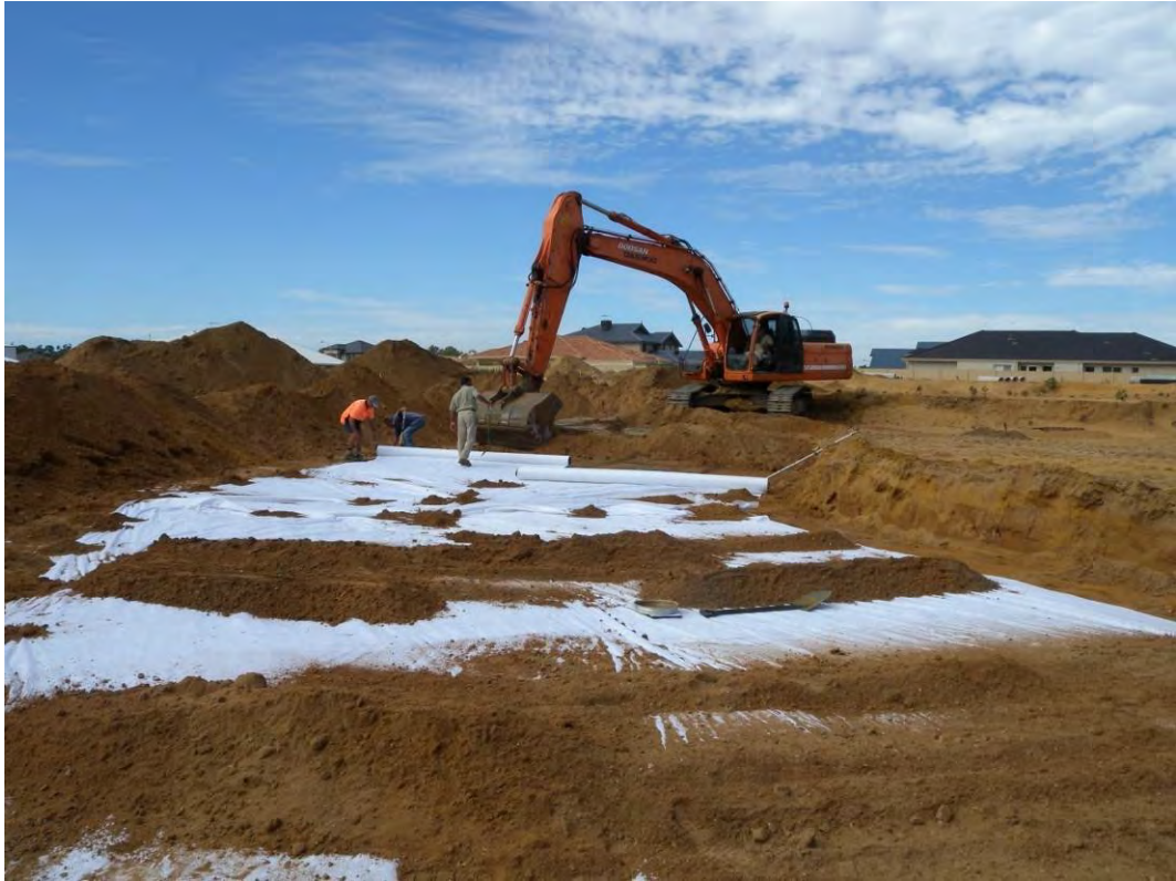
Plate A: Installation of Geotextile Barrier
