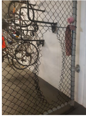
Image 1: Chain-link mesh fencing is not suitable for a bike cage (Optima 2018)
