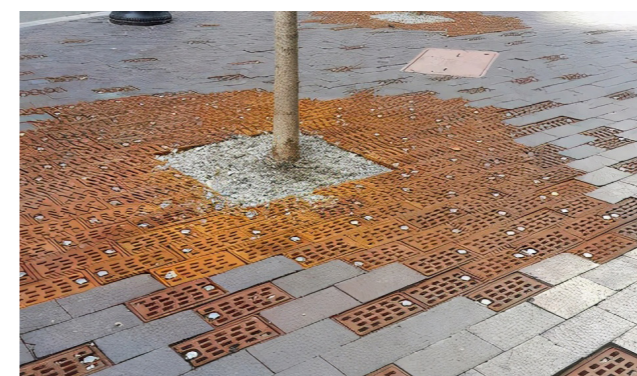
Permeable paving improve growing conditions, allow for stormwater infiltration and reduce urban heat
