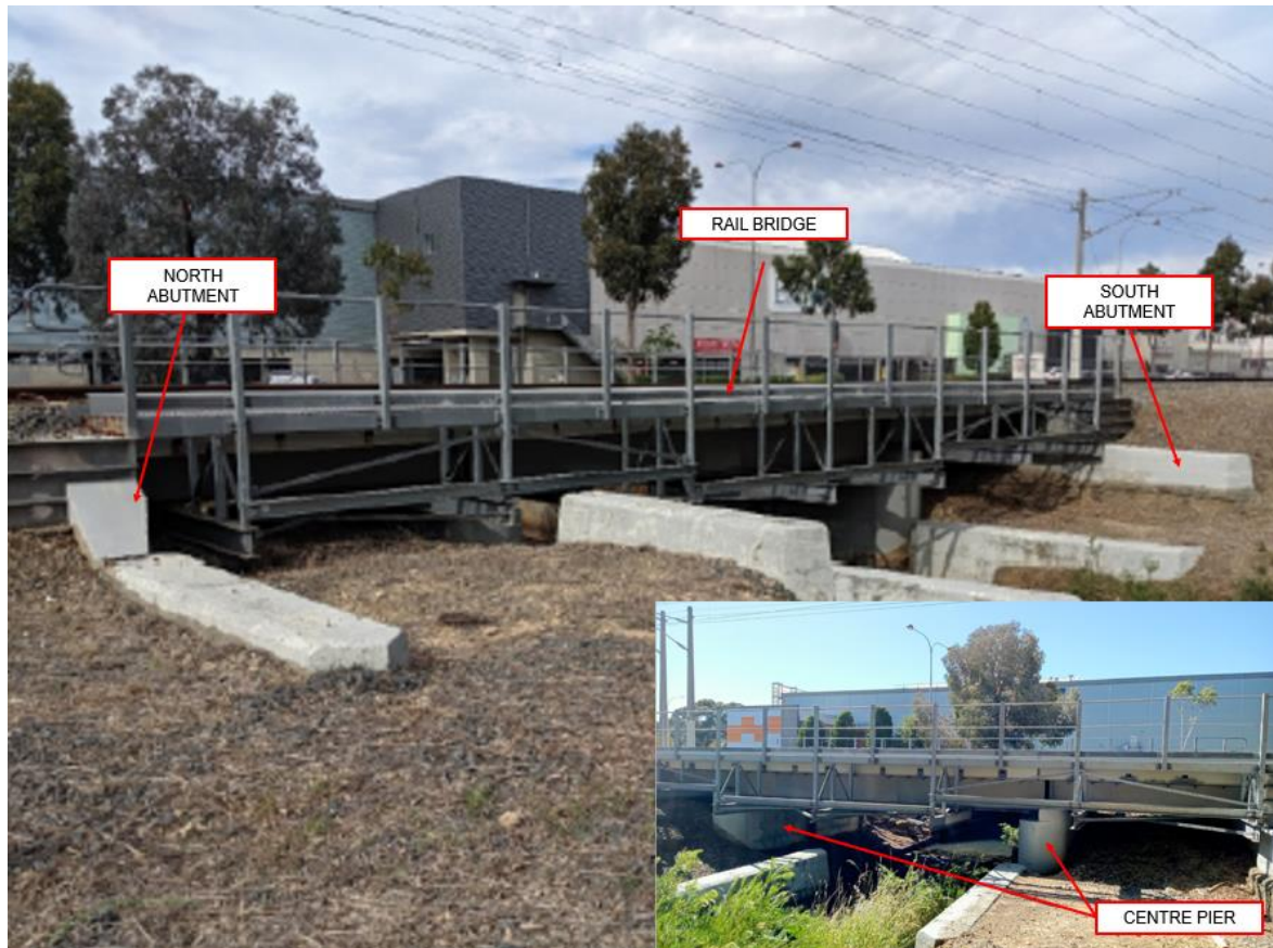
Figure 10: Neerigen Brook Bridge Demolition Areas
