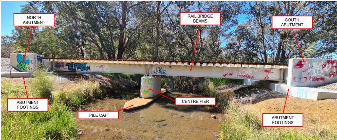
Figure 9: Wungong Brook Bridge Demolition Areas
