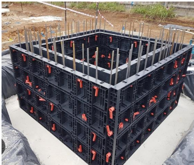
Figure 5: Example of Lift Core Formwork Systems
