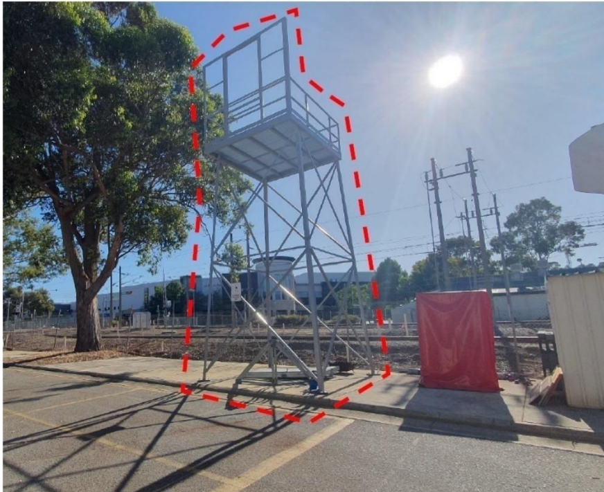
Figure 8: DFES Training Tower Demolition Areas
