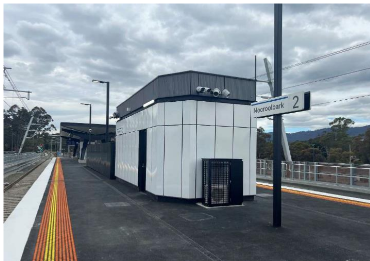
Figure 9: Example of Prefabricated Building
