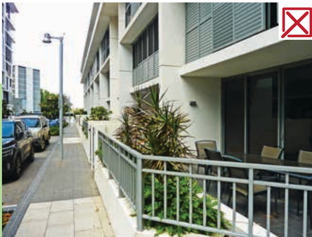
Photo 2.21 Fence design with sparse landscape and lowered courtyard may lead to a feeling of exposure for occupants.
