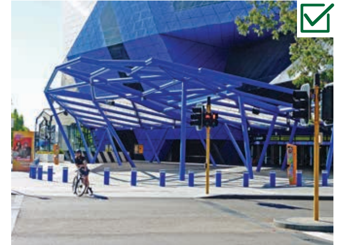
Photo 2.32 Low bollards and semi-structural bollards are used to protect the entrance of the RAC Arena.
