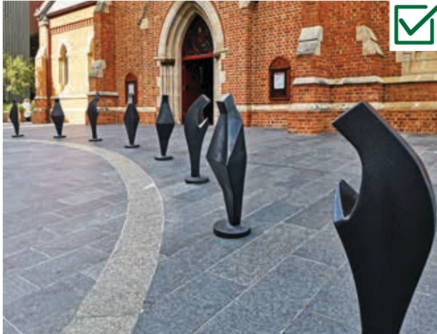
Photo 2.30 Specially designed bollards compliment the religious architecture and protect the entrance area from hostile vehicles.
