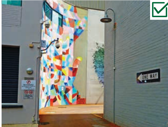
Photo 2.7 CCTV cameras and lighting improve safety for laneways that have both day and nighttime uses.
