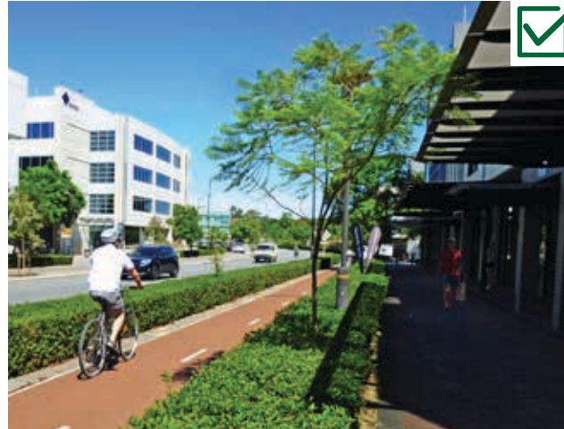
Photo 2.19 Clear demarcation of pedestrian and cyclist movement supports shared use. The different paving and colour enhance legibility.
