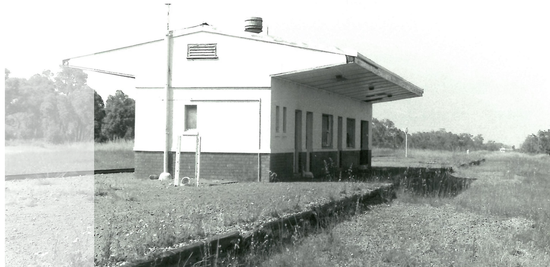
The old Byford railway station, shortly before demolition (1987). Photo: Ian L. Boersma
