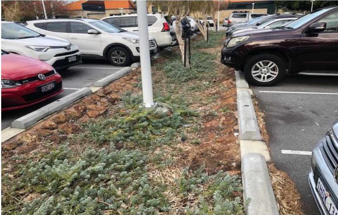
Figure 7.9. Typical Carpark Bio Swale Treatment Area
