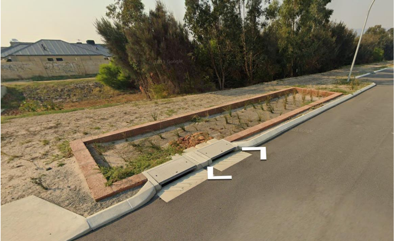
Figure 7.6. San Simeon Blvd – Median Swale Treatment
