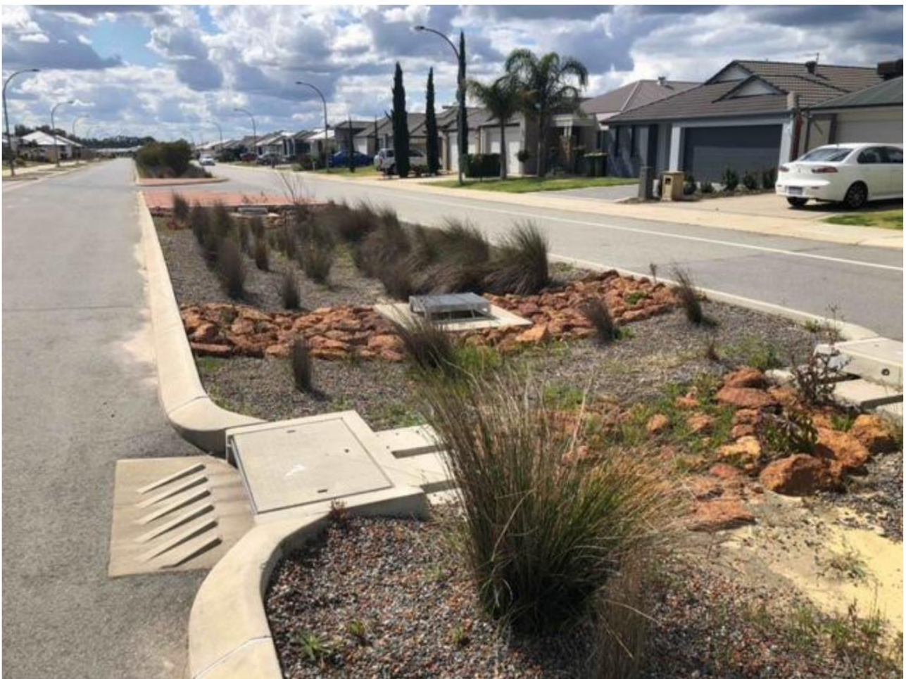
Figure 7.5. San Simeon Blvd – Median Swale Treatment
