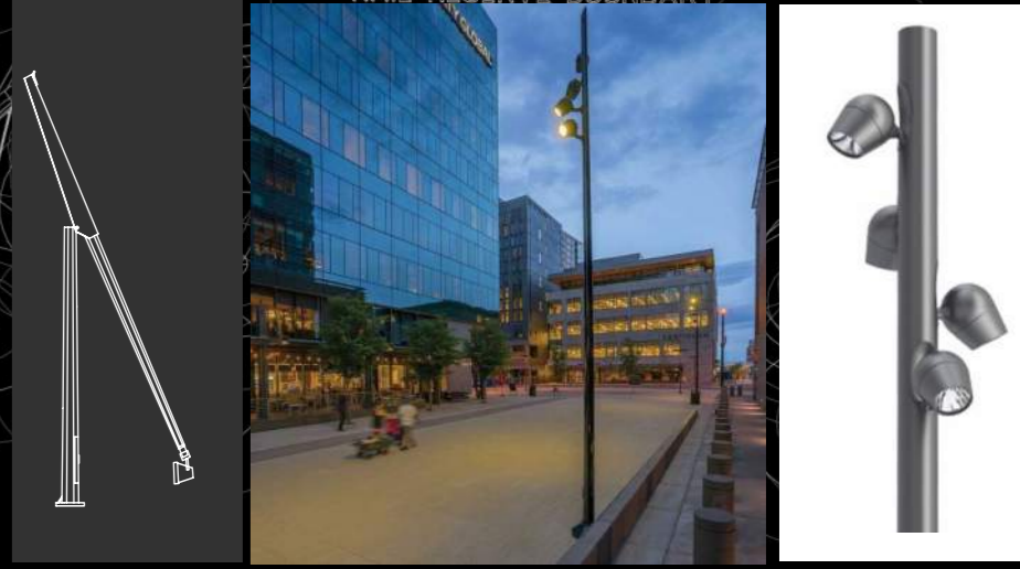
CLUSTER OF OUTDOOR SPOT LIGHTS FIXED TO 8M SEESAW TYPE POLE TO ILLUMINATE PLAZA AREAS
