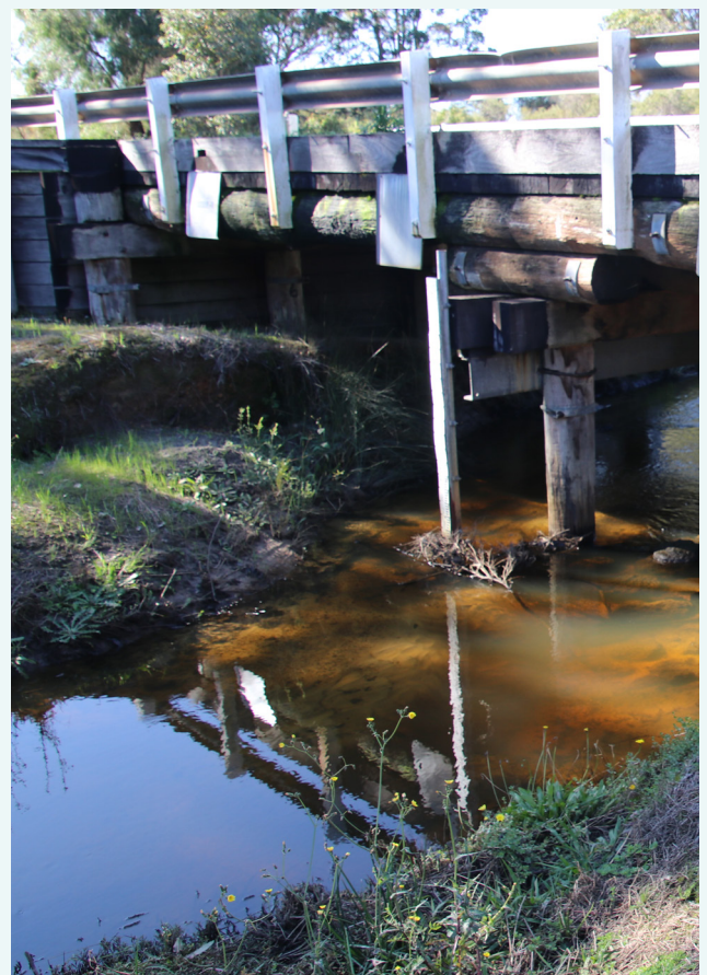
The Glenarty Road Bridge on Glenarty Creek, August 2019.
