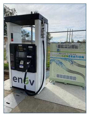
Figure 3.18 Vehicle Hydrogen Refuelling Skid
