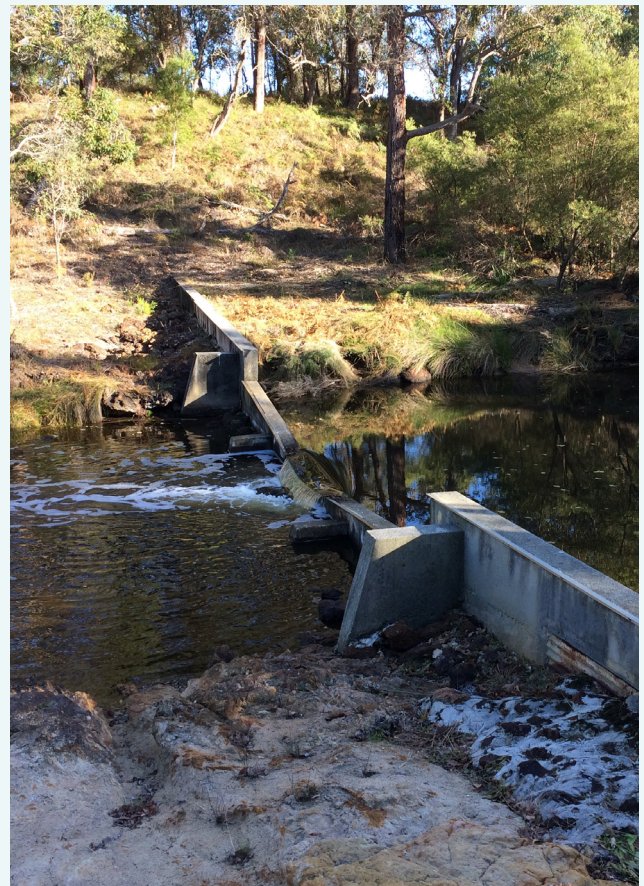
The Kalgan River weir during low flow, May 2018.
