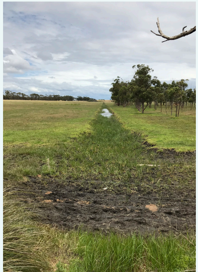
A paddock drain. Drains like this are used to help prevent water ponding in paddocks, November 2020.
