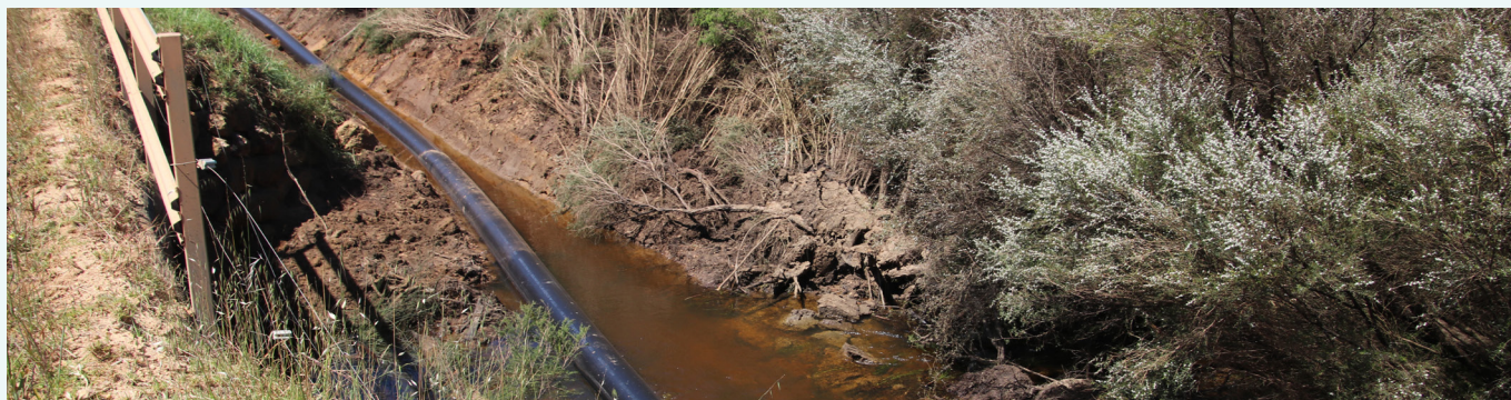
An irrigation pipe being buried at the McLeod Creek sampling site, November 2018. This pipe provides irrigation water from the dam upstream of the Rushy Creek sampling site.
