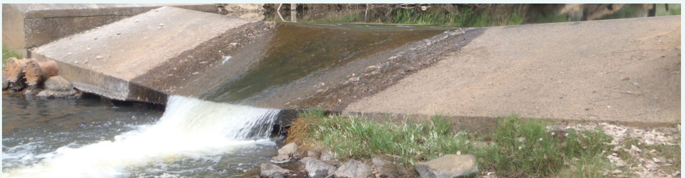
Low water levels at the Preston River sampling site, November 2018.
