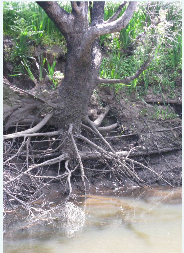
Erosion and slumping along the banks of the Preston River, October 2009.
