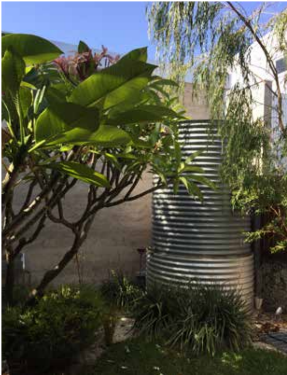
Photo G1.4a Compact rainwater tanks can be neatly located within the primary garden area
