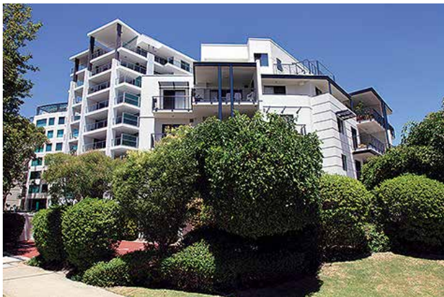
Dense landscaping provided between the building and the street, however, visual surveillance is maintained. The landscaping is a key feature in defining the building.
