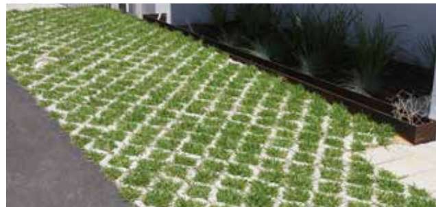
Photo G1.4b Permeable pavers planted with hardy waterwise plants can provide trafficable areas
