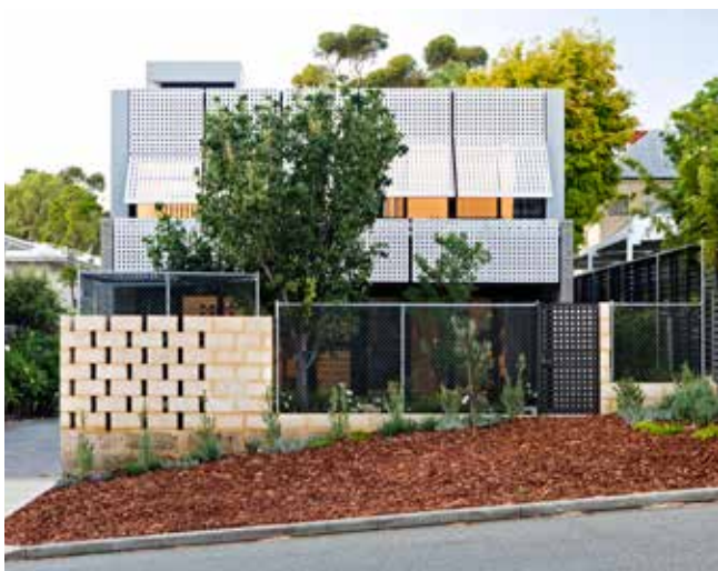
Photo G1.2d Provision of trees in the street setback area enhances the streetscape character and softens built form (PC)
