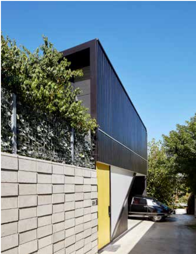
Photo G2.8a This ancillary dwelling is built above the garage (Fonzie Flat) and is independently accessed from the laneway (PC)
