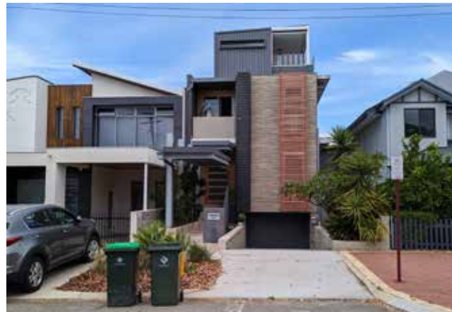
Photo G3.2a Where narrow lots are proposed it may be appropriate for building heights to increase. This example sets back the third storey to minimise impact on adjoining properties
