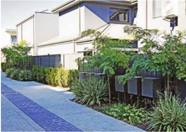
Photo G2.5c Landscaping effectively screens the essential service utilities in this communal street, whilst maintaining convenient and safe access
