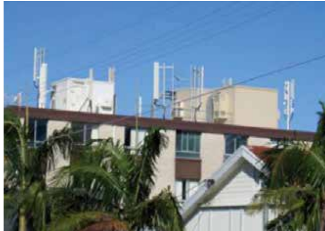
Rooftop plant and infrastructure dominates appearance of the building.
