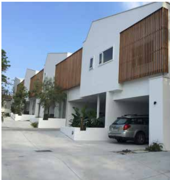
Photo G3.5a This row house development steps down with the slope of the site
