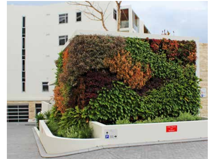
Photo G1.2b Planting on structure – a green wall at the entry to an apartment building
