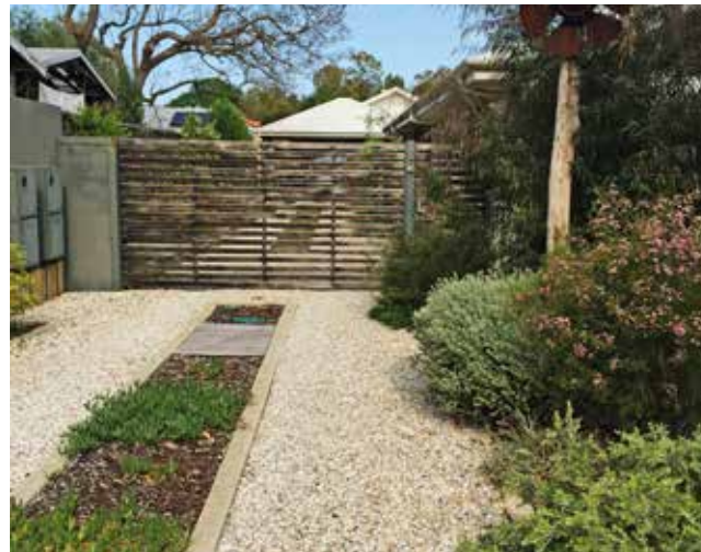
Photo G3.7b This shared driveway space has been designed and constructed to be fully permeable, and includes planted areas and a gravel surface
