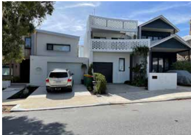
Photo G3.4a When proposed in a coordinated manner, two storey boundary walls support efficient design and construction outcomes with minimal impact on adjoining properties
