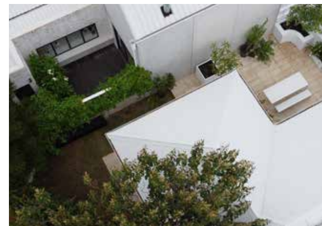
Photo G3.1a This grouped dwelling development with a retained dwelling has carefully managed site cover to create useable outdoor spaces around each house (PC)
