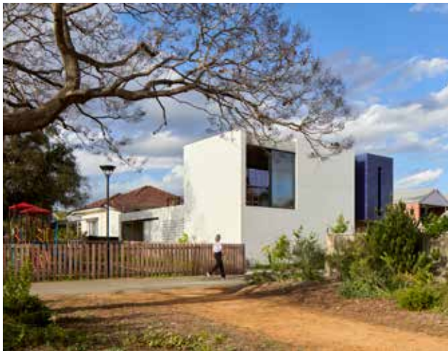
Photo G3.9a This dwelling is designed to reduce the impact of development overshadowing primary garden area of adjoining lot (PC)
