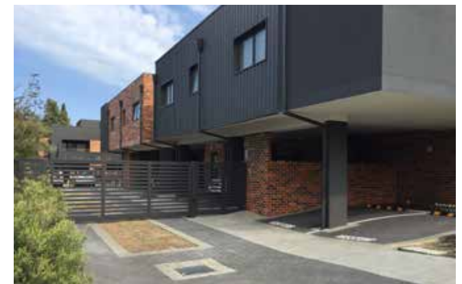
Photo G2.3b The visitor parking is easy to find and is located outside the development's security gate for accessibility
