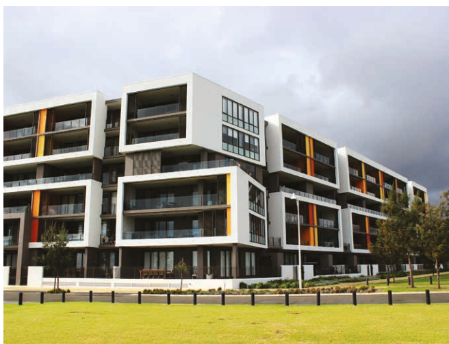
Photo 4.10a A 'twist' at the corner creates an interesting play on the strong geometrical lines of the façade, highlighting the corner of the building.
