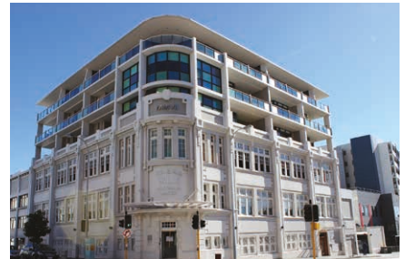
Photo 4.13a Additional levels of apartments reinforce characteristics of the existing heritage building while remaining modern and distinct.
