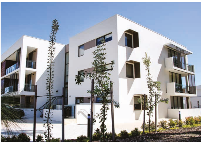
Photo 4.1e Simple sun shading device can be effective in minimising heat and glare. (PC)
