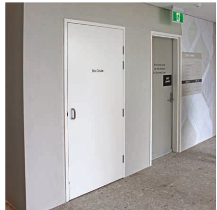
Photo 4.17b Communal waste facilities associated with circulation cores at each floor make waste handling convenient for residents.
