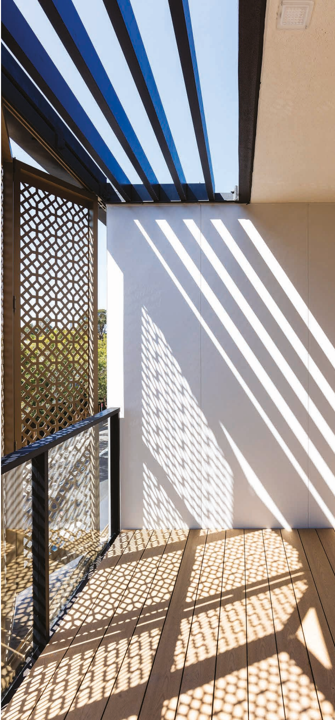
Photo 4.2a Sun screen and pergola structure provide shade and at the same time allow for natural ventilation. (PC)
