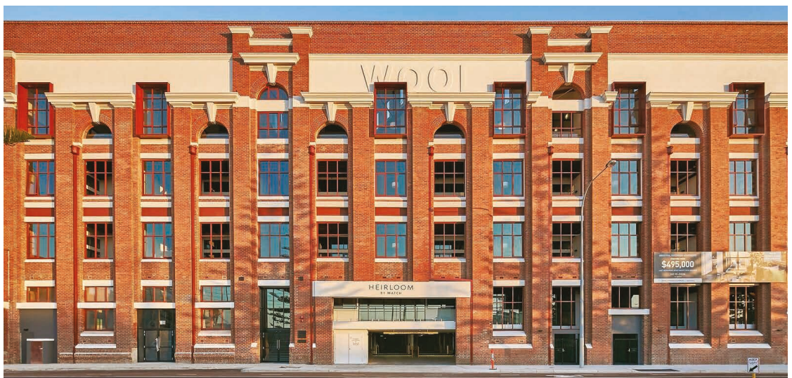
Photo 4.13c This adaptive reuse project protects the heritage and character of the old Woolstores building and turned it into 183 apartment units. (PC)
