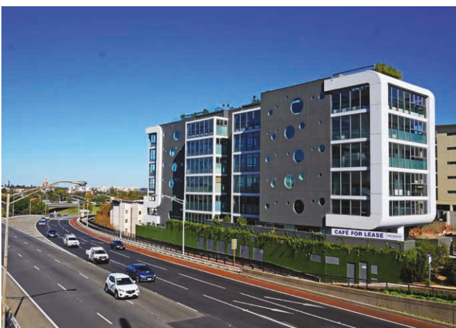
Photo 4.7b Development next to a freeway needs sufficient noise abatement measures such as those listed in DG 4.7.3. (See also Photo 4.7c, showing some of the noise reduction features in the same building).
