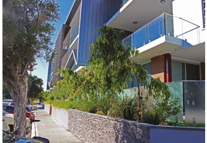
Photo 3.6e The raised planter and landscaping enhance the privacy of these ground floor apartments, improve the public domain interface and at the same time contribute to the greening of the streetscape.
