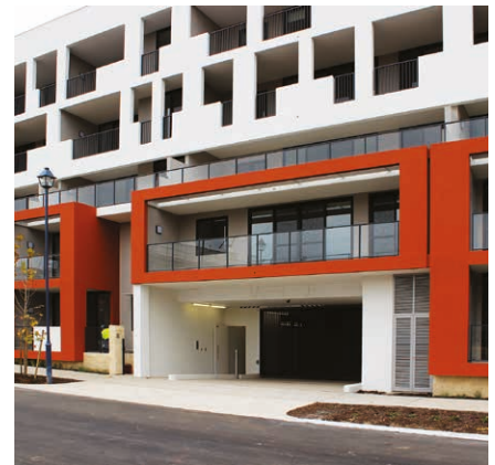
Photo 3.8a This clear vehicular access has a low impact on the streetscape and integrated well into the façade design of the building.
