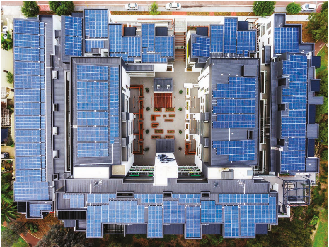
Photo 4.15a This apartment development fully utilises the roof with the installation of photo-voltaic arrays to supplement the power consumption of the dwelling units. (PC)
