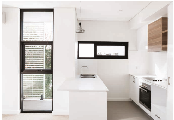
Photo 4.2b, c & d (From top) Louvre, casement and awning windows are preferred to sliding windows as the latter provide limited opportunity for the control of breeze. (PC)
