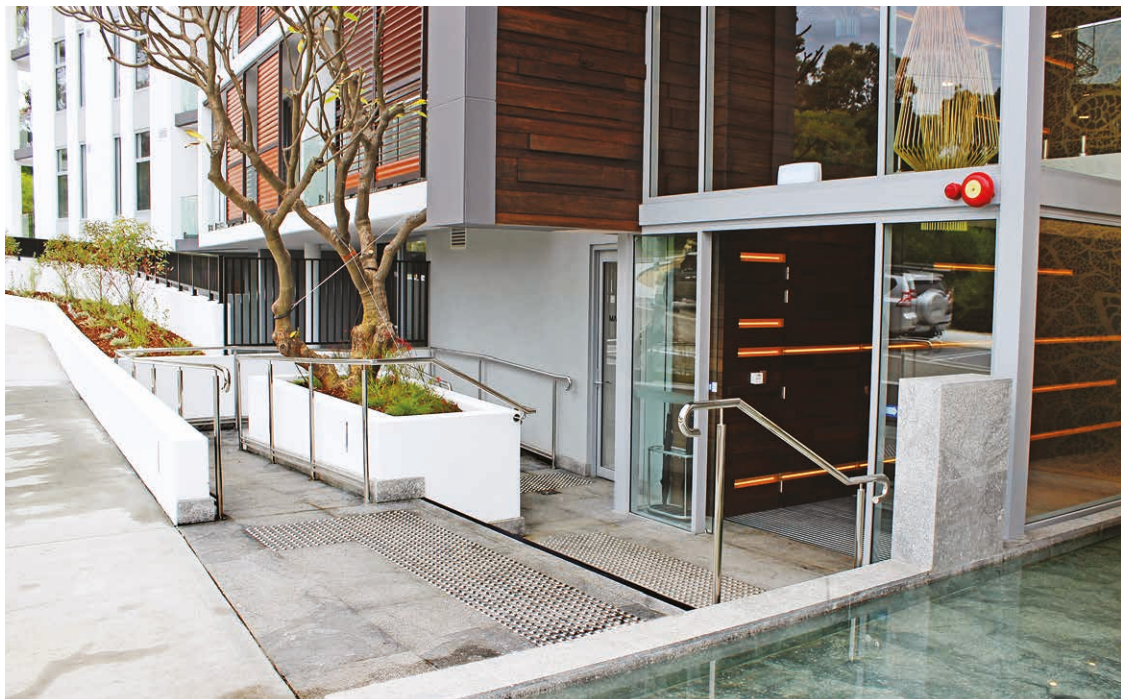
Photo 4.9a A step-free entrance is provided in this apartment block, taking into consideration universal access.
