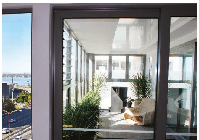
Photo 4.7c Sliding sash glazing and louvre windows in this wintergarden enables modulation of enclosure and openness, at the same time reduces the impact of traffic noise from the adjacent freeway. Installation of special noise absorbing ceiling material also helps in noise reduction.
