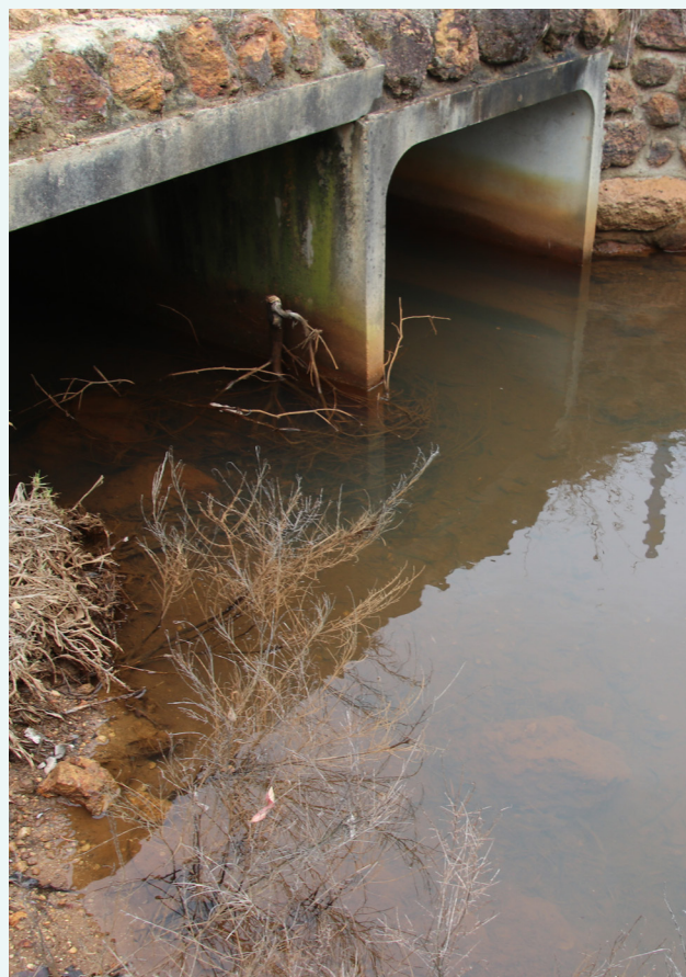
The culverts through which Turnwood Creek passes under Fisher Road, October 2019.
