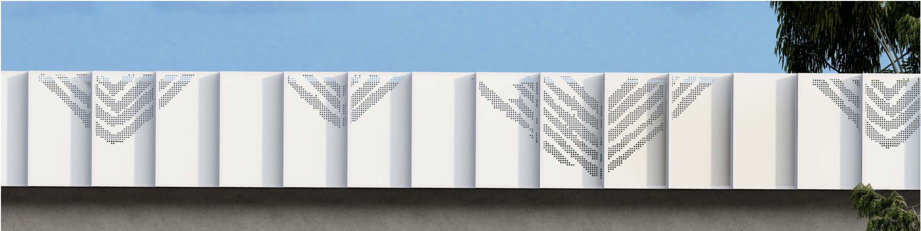
Lower Intensity Pattern Linewide (4.6% Perforate)
