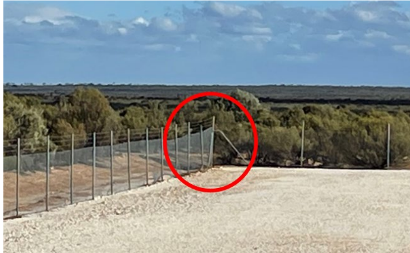
Disposal Cell 97NRT01 South End Prior to Maintenance
