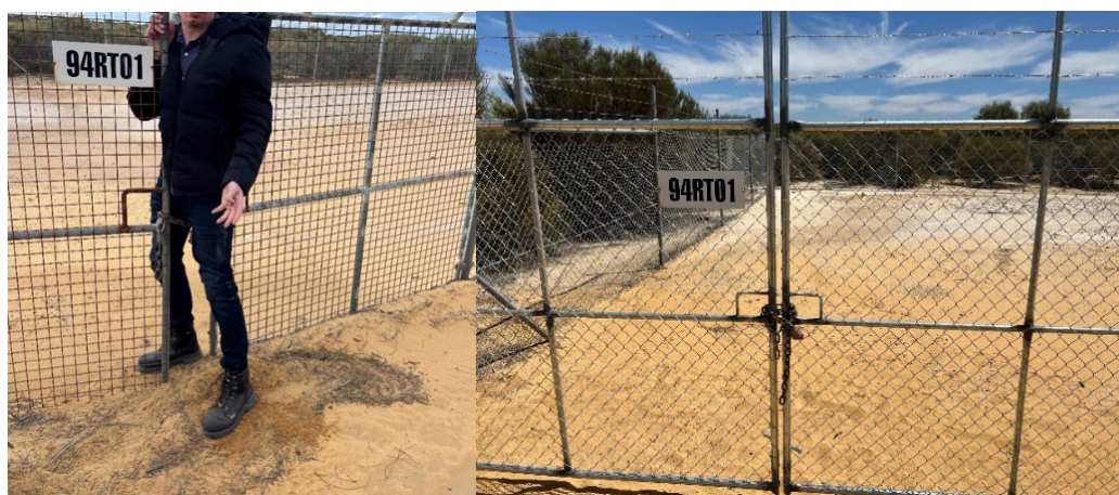
Disposal Cell 94RT01 Gates Before and After Maintenance
