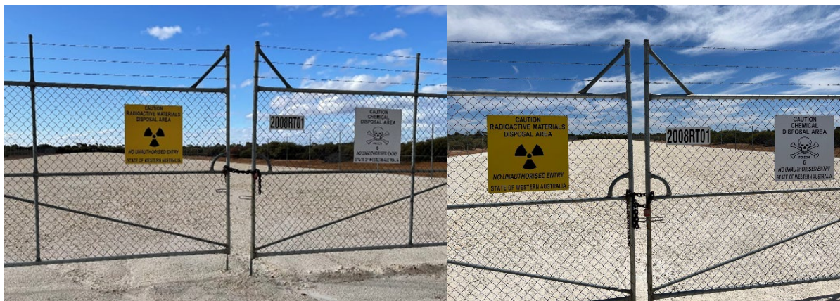
Disposal Cell 2008RT01 Gates Prior to Maintenance After Maintenance
