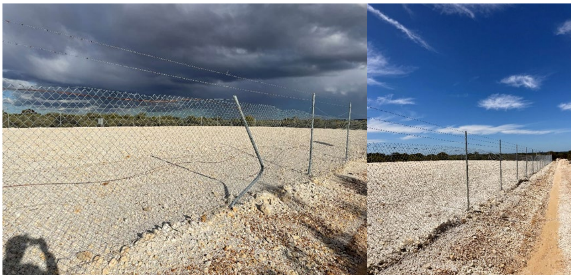
97NRT02 Disposal Cell Fencing Prior to Maintenance
