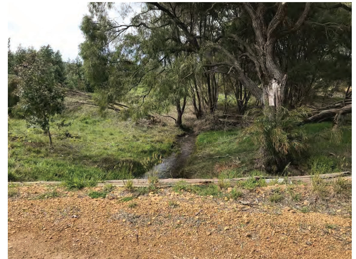
Plate 1: Condition of main waterway at existing crossing location
