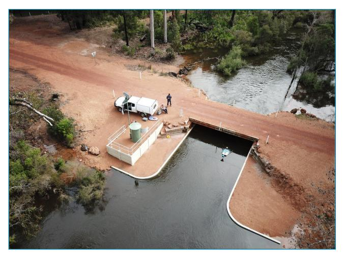
Figure 4 New gauging station infrastructure on Manjimup Brook is allowing us to permanently measure streamflow while better enabling fish passage.
