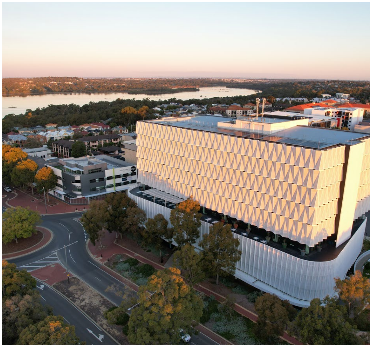
The department's Prime House head office. Picture: Davin Storey
