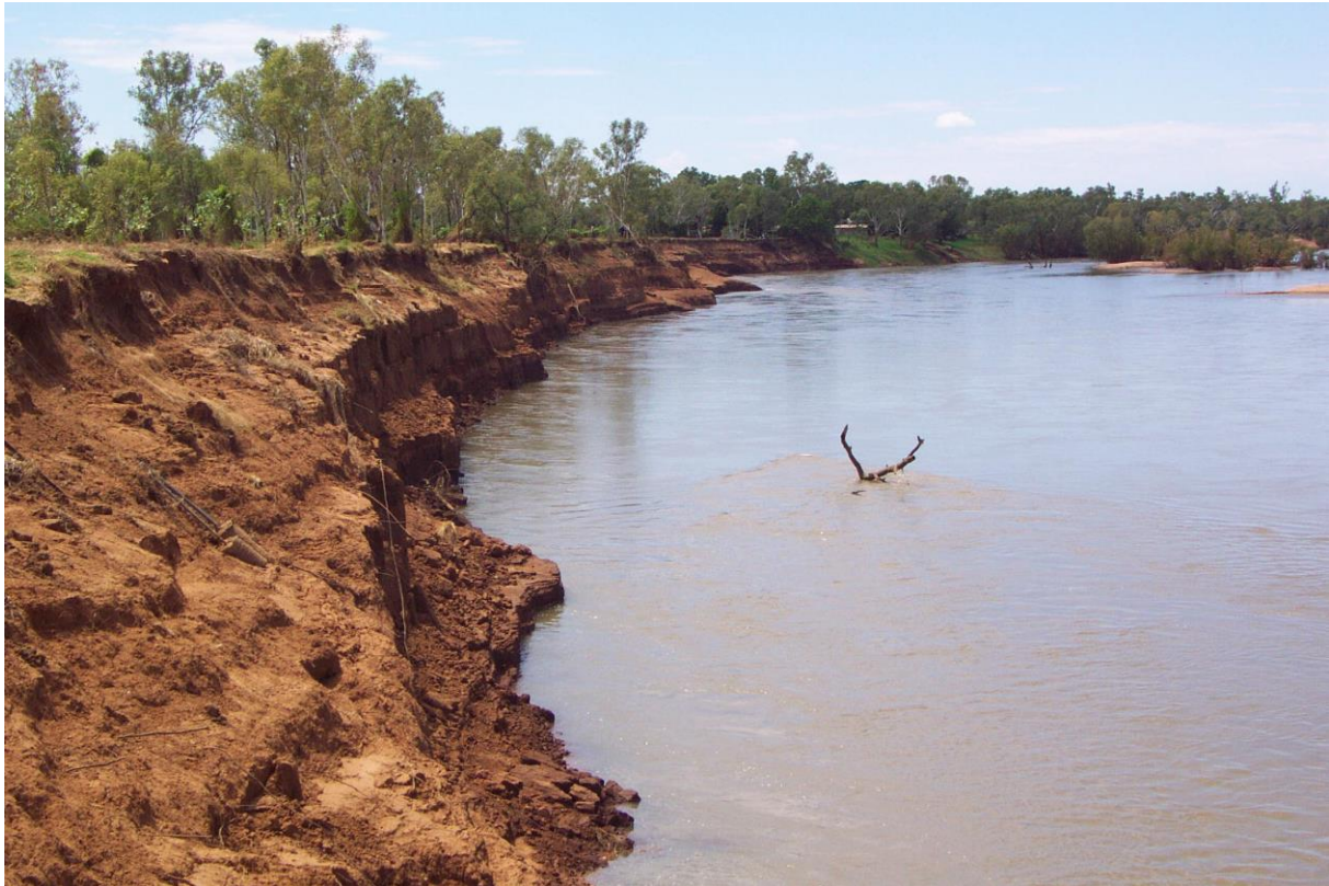
Figure 43 Riverbank erosion near Fitzroy Crossing following flow in 2002
