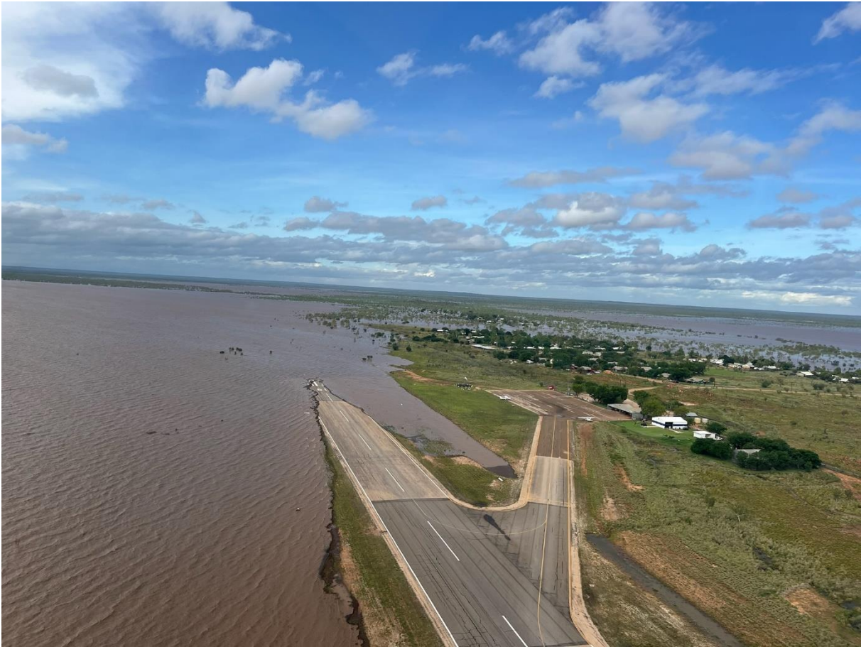
Figure 34 Floodwaters surrounding Fitzroy airport in January 2023
