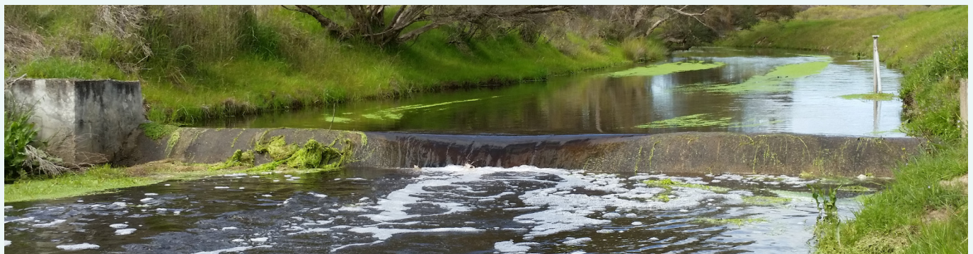
The weir at the Coolup South Main Drain sampling site, August 2016.
