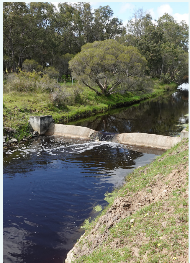
The weir at the Coolup South Main Drain sampling site, September 2018.
