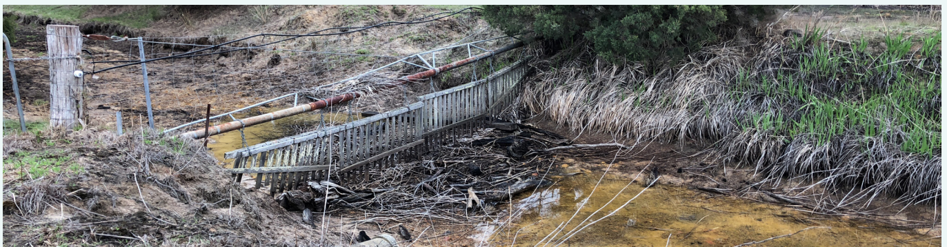
Woody debris caught on a trash rack in Cuppup Creek, July 2018.
