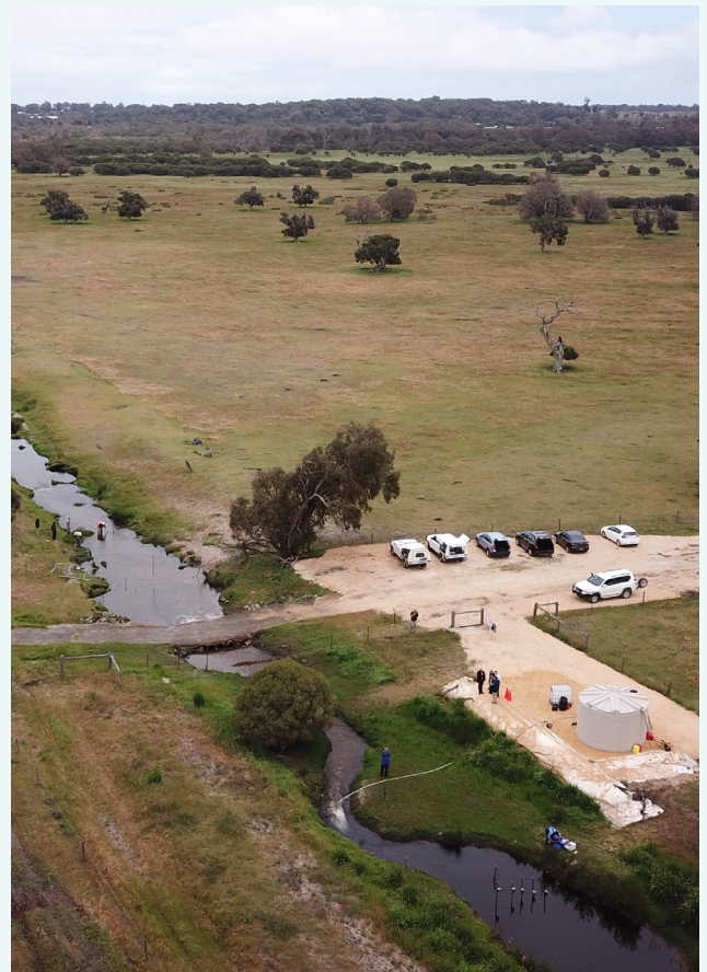
Aerial view of a drainage water treatment trial site in Punrak Drain. Phosphorus-binding clay is being added to the drain to remove phosphorus from the water, October 2017.
