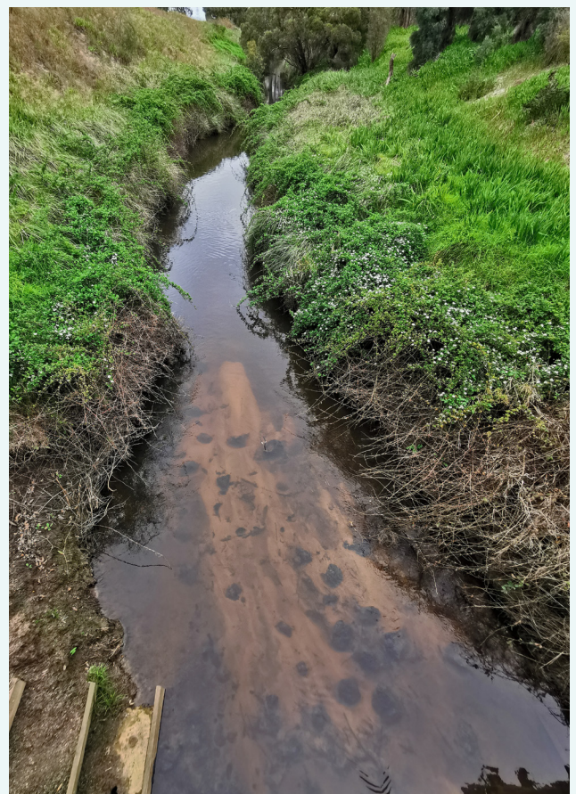
Warooona Drain. Note the sand slug in the bottom of the drain. This is from erosion further upstream with the sand being deposited in slower-moving sections of the drain like this one, September 2020.
