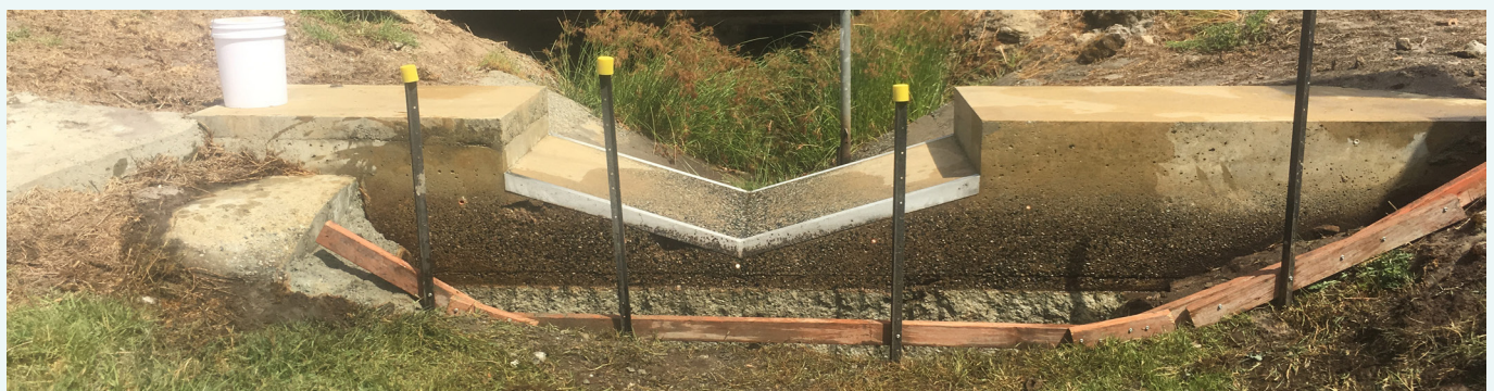
Looking downstream at the weir at the Gull Road Drain sampling site when it is dry, March 2019.
