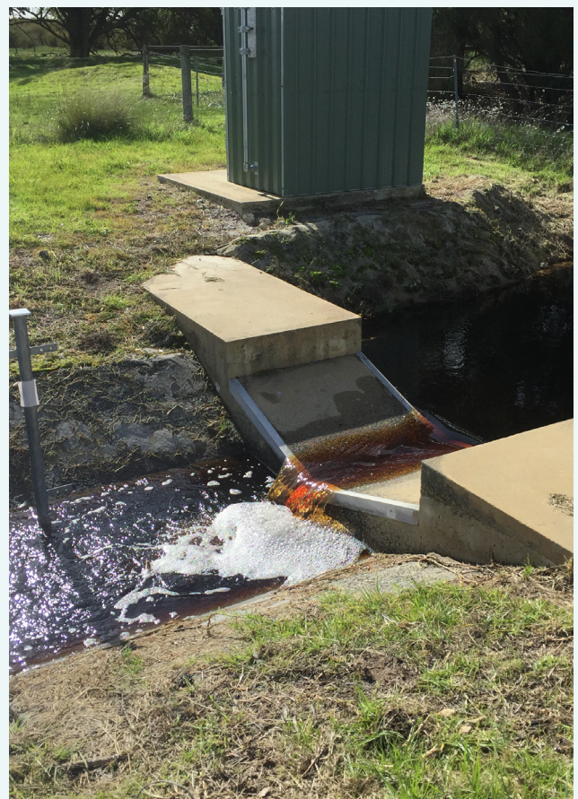
The weir at the Gull Road Drain sampling site, July 2018.
