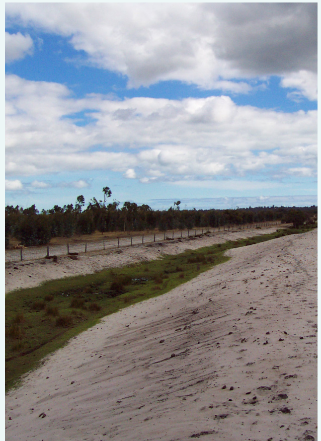
A drain in the Gull Road Drain catchment. Note the sandy banks which will easily erode if stock walk along it or water levels are high, April 2002.
