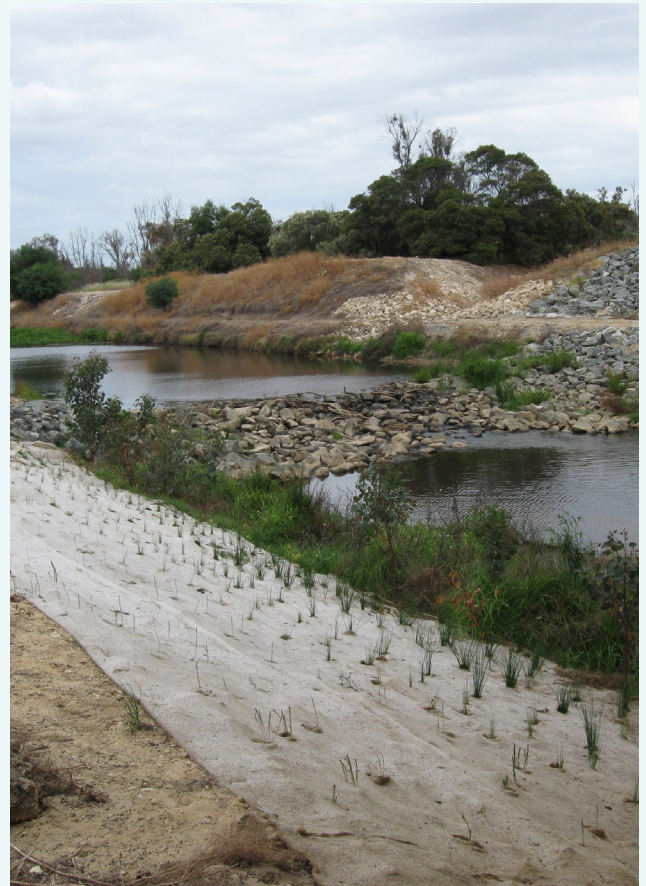
Revegetation on the bank of the Harvey River at the sampling site. This helps stabilise the banks and reduces erosion, December 2008.
