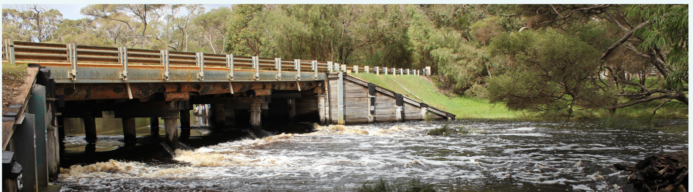
The Brennans Bridge sampling site during high flows in September.
