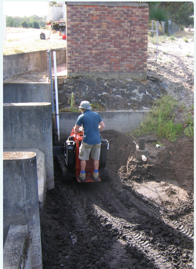
Removing particulate matter and sediments which have settled in front of the gauging station at Meredith Drain, May 2020.
