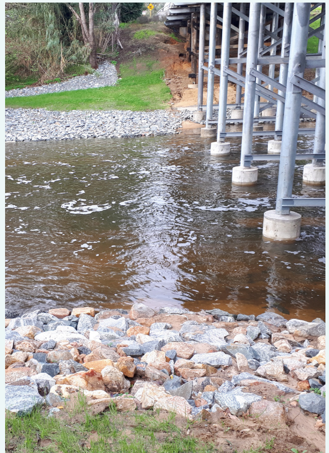
The Pinjarra Road Bridge at the Middle Murray sampling site. The rocks along the banks are there to help stop erosion, June 2018.
