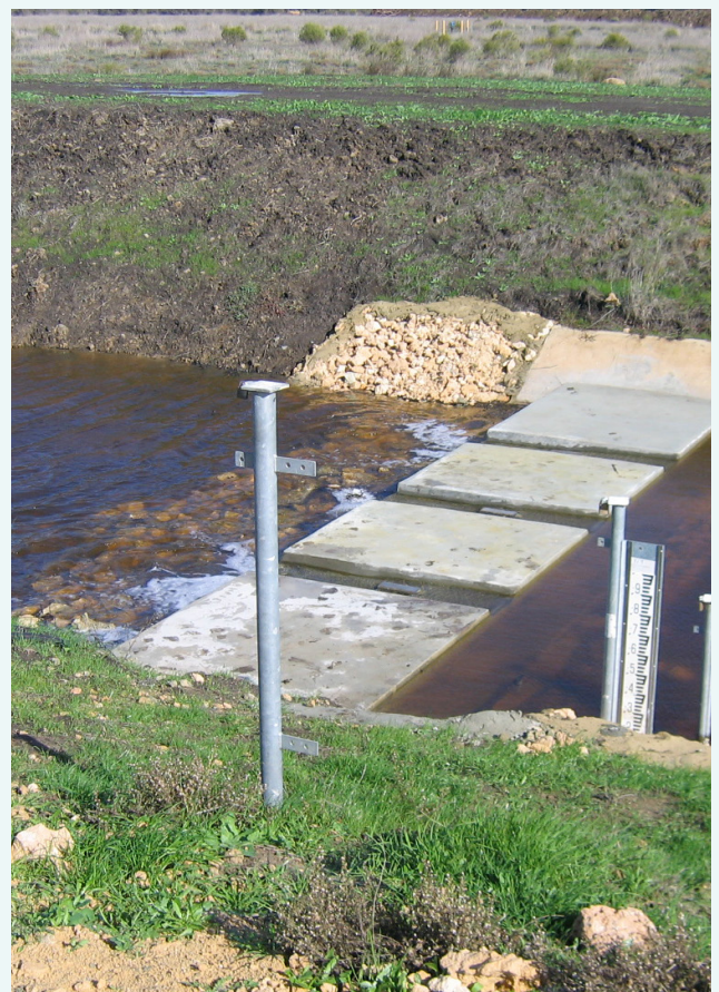
The weir at the Peel Main Drain sampling site, May 2007.
