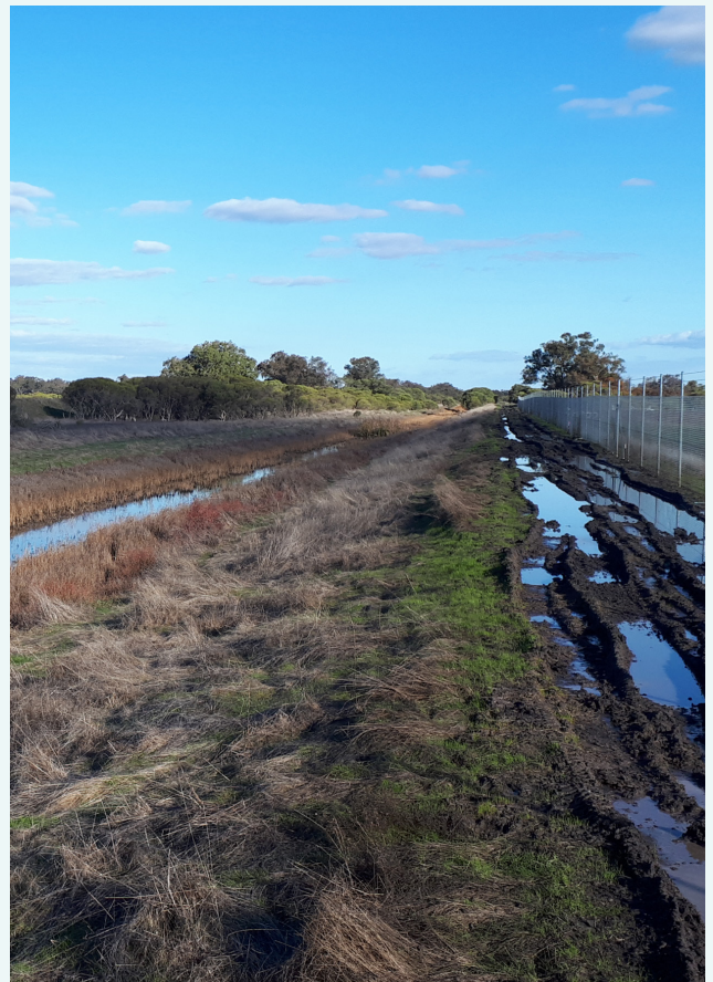
Peel Main Drain, note the waterlogging along the fenceline to the right of the photograph, June 2019.
