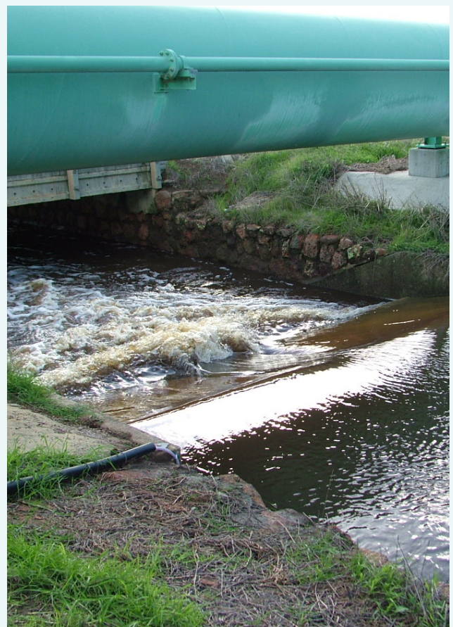
The weir at the Samson North Drain sampling site, May 2005.
