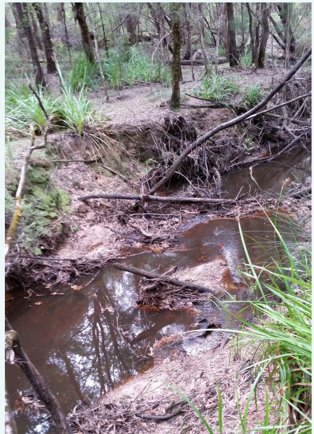
Low water levels in Scotsdale Brook, January 2018. Note the erosion of the banks.
