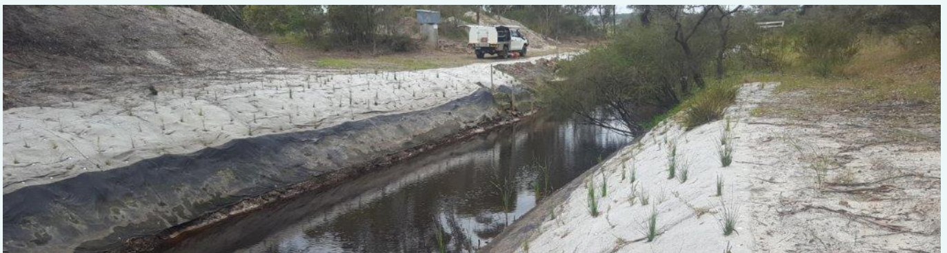
The Sleeman River sampling site after the sedimentation was removed from the channel and the banks were stabilised using matting which was planted out with native species, October 2019.
