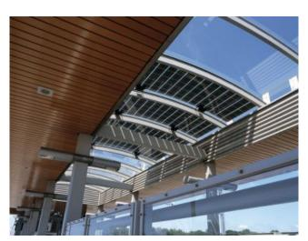
Image 43: Solar Panels Integrated into Awnings
