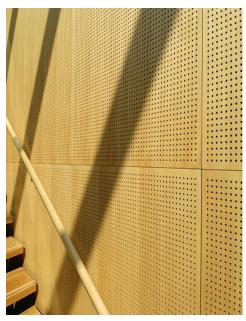
Image 21: Perforated Interior Acoustic Panel
