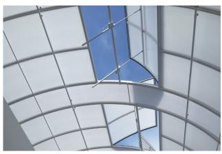
Image 14: Barrel Vault Roof Lights
