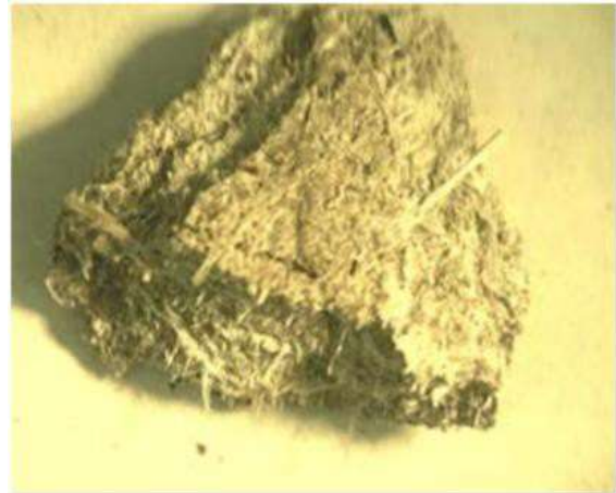
Cement based sheeting with white asbestos
