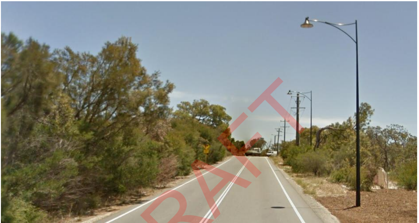
Figure 17 Rowley Road view to west (Source: Google Maps)
