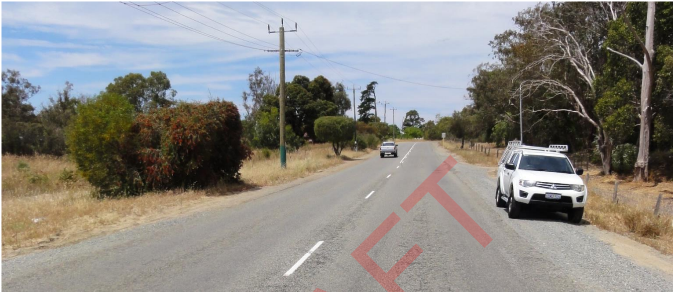
Figure 25 Mandogalup Road view to south (Source: Flyt)
