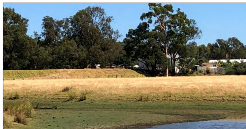
View across floodplain to existing levee bank
