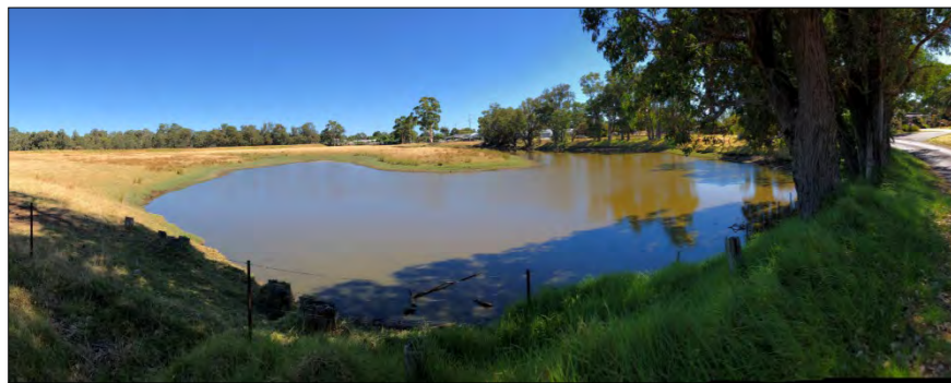
Portion of existing floodway on private property
