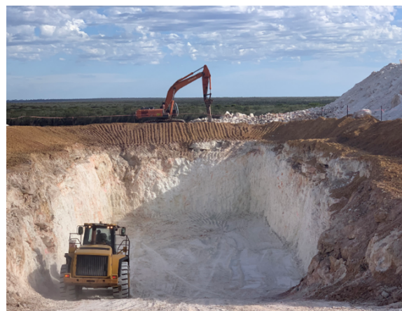
Excavation of the 2020NRT01 Disposal Trench
