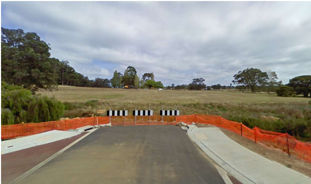
Figure 2.4: Access link prepared off Rapids Landing Avenue Source: Streetview
