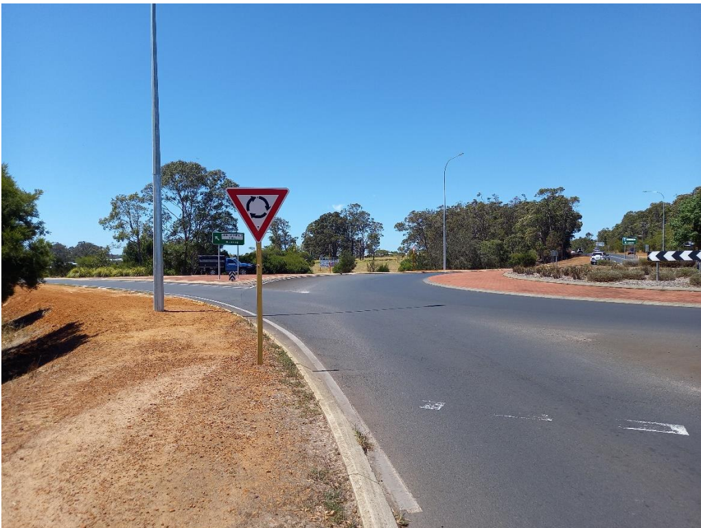
FIGURE 8: VIEW INTO SITE FROM BUSSEIL HIGHWAY ROUNDABOUT
