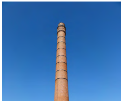
Remnants of the Robb Jetty Chimney are still in place today
