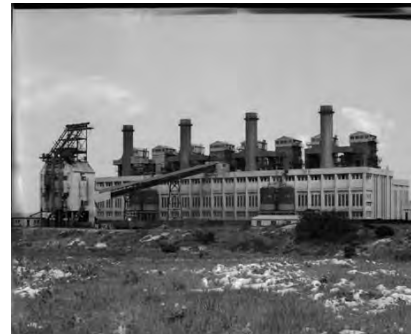
The South Fremantle Power Station in operation (State Library of WA)
