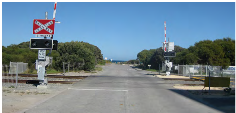
Figure 22_Freight rail in the Cockburn Coast & South Beach
