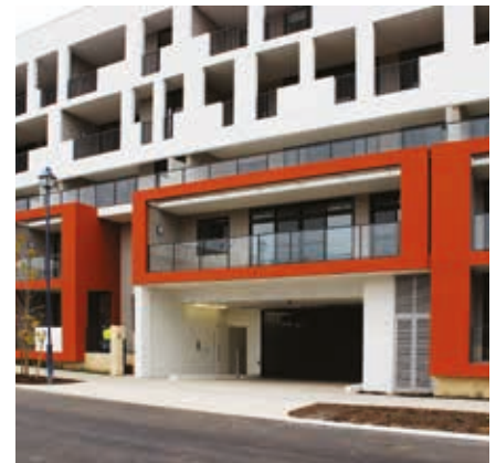
Photo 3.8a This clear vehicular access has a low impact on the streetscape and integrated well into the façade design of the building.
