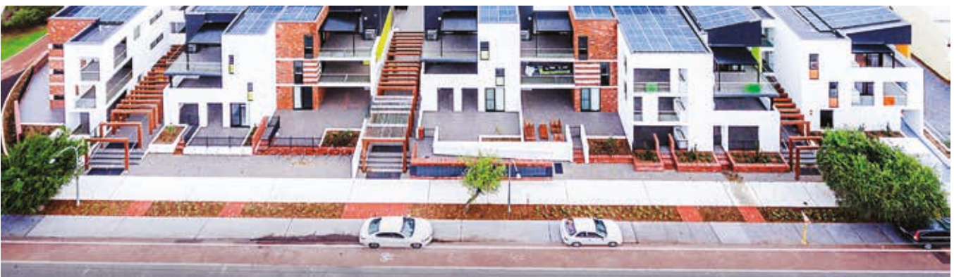
Photo 3.6h Some good public interface elements are demonstrated here: the three street entries points are clearly legible, one of them has universal access; change in level between footpath and front courtyards for privacy allowing for largely permeable fencing; upper level balconies and windows overlook the street and public domain areas ensure public surveillance; mix of textures and materials provide pedestrian interest; mail boxes and bike racks are well integrated along front fences; landscaping provision is generous and enhances the layout design. (PC)
