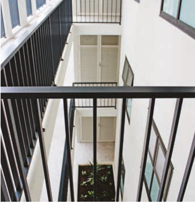
Photo 4.5d Communal walkway is separated by a void from dwelling windows to provide some degree of privacy.
