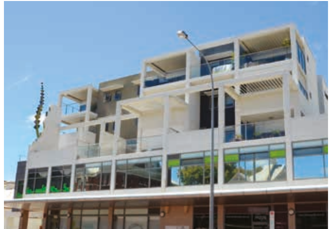
Photo 4.1d Shading and glare-control measures help to moderate solar gain for west-facing windows and balconies, including operable roof louvres to optimise sunlight and shelter.
