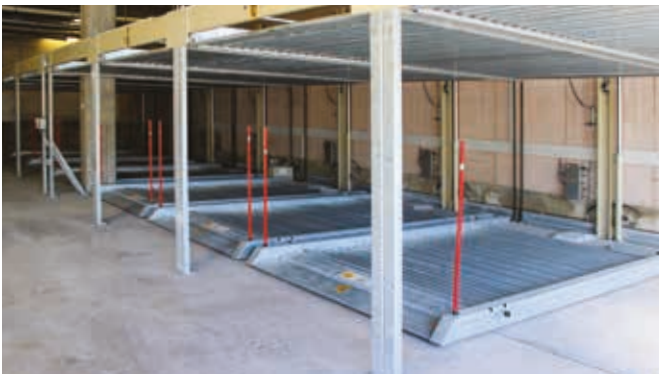
Photo 3.9d Car stackers can provide a space-efficient solution.
