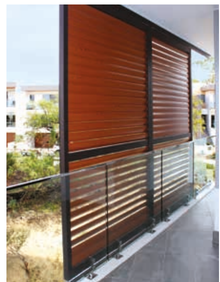
Photo 4.4d Operable shutters can be used to control sunlight and wind, as well as enhanced privacy.
