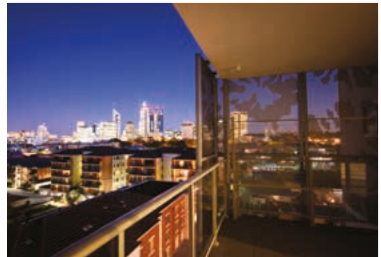
Photo 4.4b Balconies can enhance the amenity of the residents by providing extra space and views. (PC)
