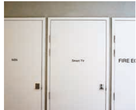
Photo 4.18b This apartment is fibre-to-premises ready.
