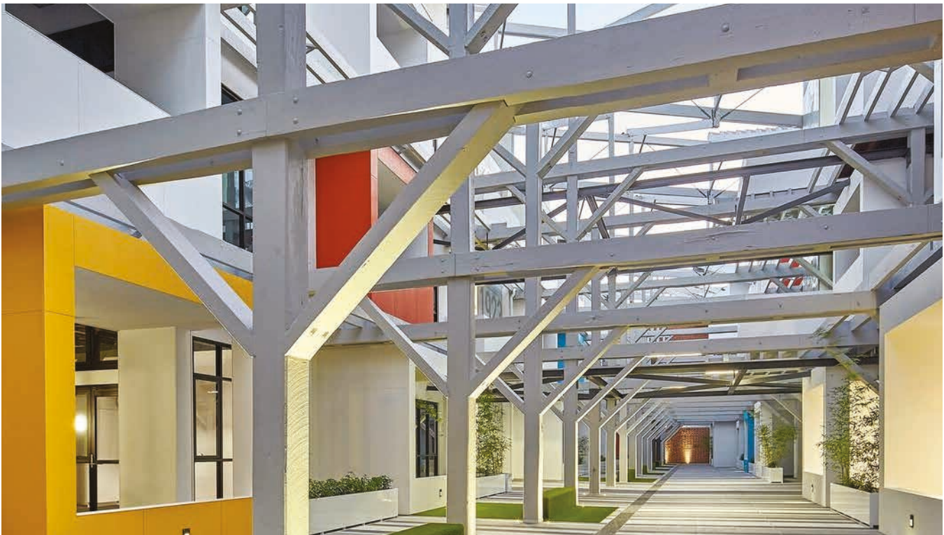
Photo 4.5f The roof and floors in the middle section of this adaptive reuse of a heritage building have been removed to allow for better natural ventilation and light to reach the circulation area. (PC)
