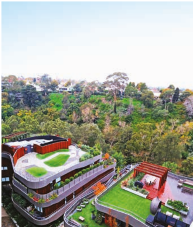
Photo 4.11a Open space, landscaping and other amenity provisions are maximised on these roof and balcony spaces.
