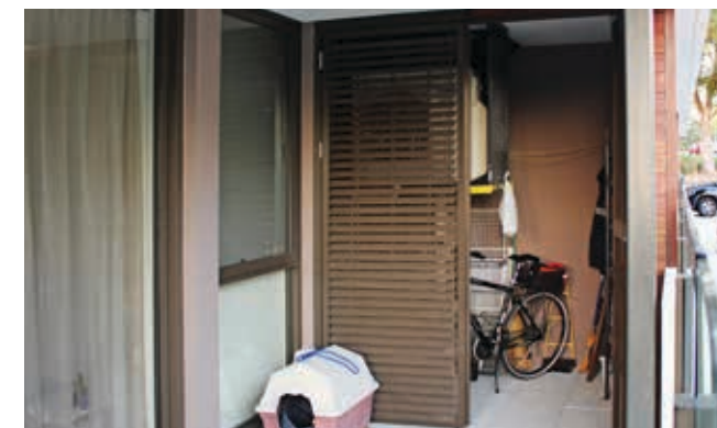
Photo G2.1b and c This storage area has been neatly integrated into the design of the balcony, is conveniently located, is of useful size and proportions, weatherproof, and screened from view
